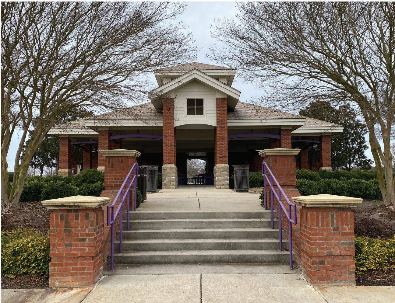
NRC EXISTING FIELD HOUSE
