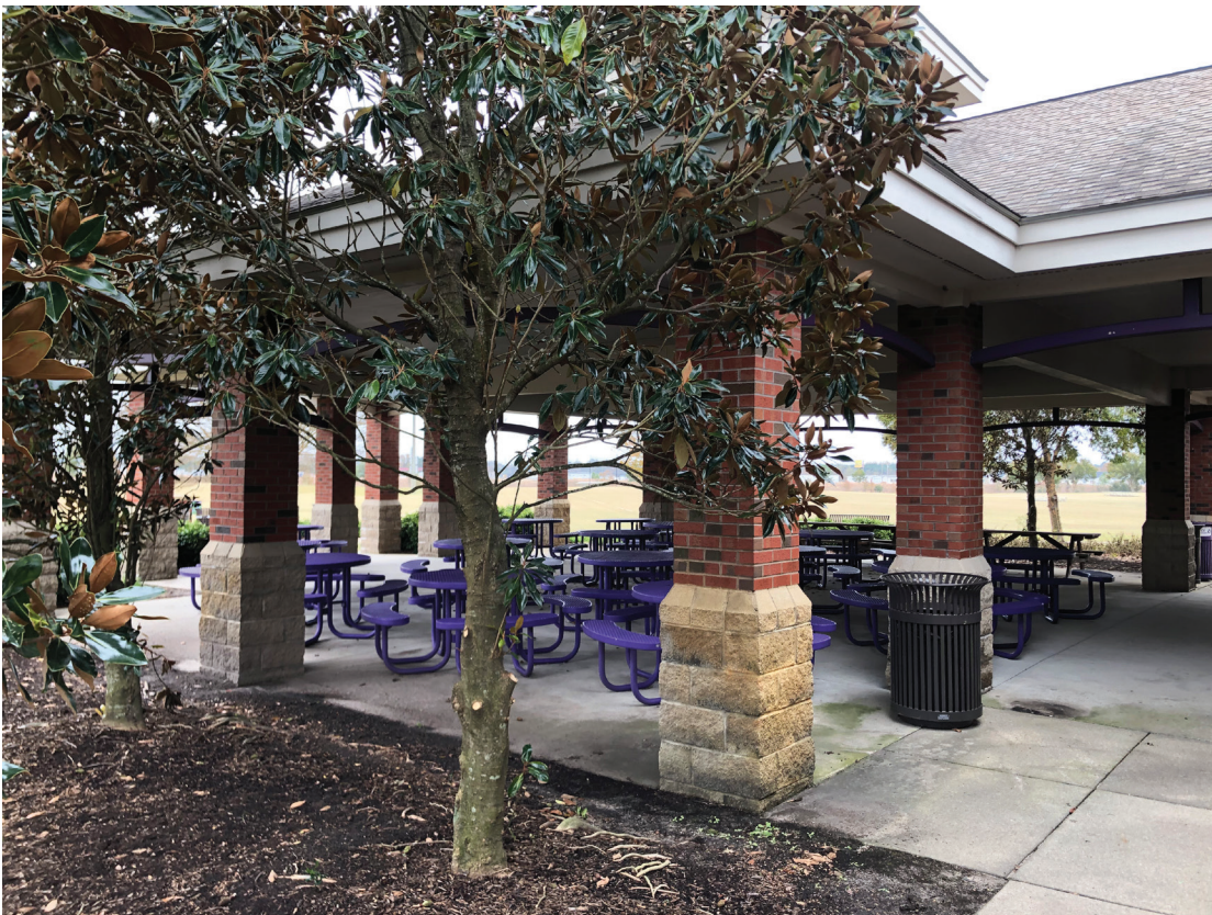
NRC EXISTING PAVILION
